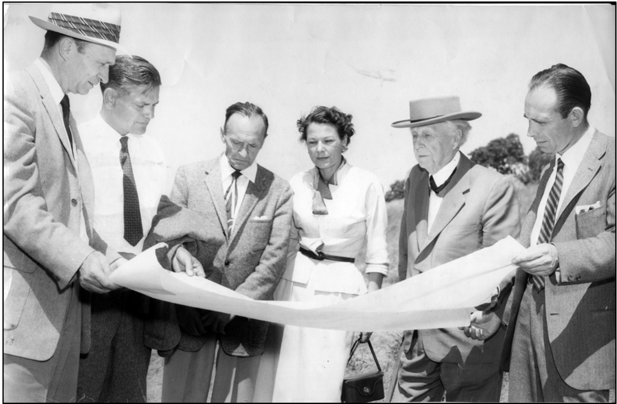
Figure 14. August 1, 1957 Frank Lloyd Wright visits site and studies a topographical map for future Marin County Civic Center; Marin County Planning Director Mary Summers at center, Frank Lloyd Wright, right of center, Aaron Green, Marin City Public Housing Architect, far right (three gentlemen at left unidentified) Source: Aaron Green Archive
